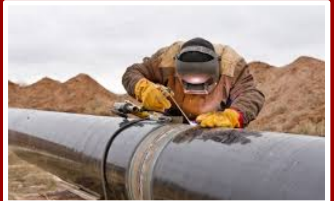
Pipeline Construction (Flow-line Manifold Fabrication etc.)
