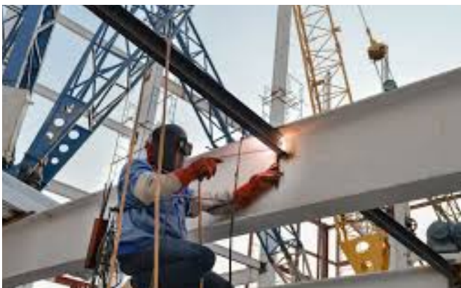
Structural Steel Fabrication
